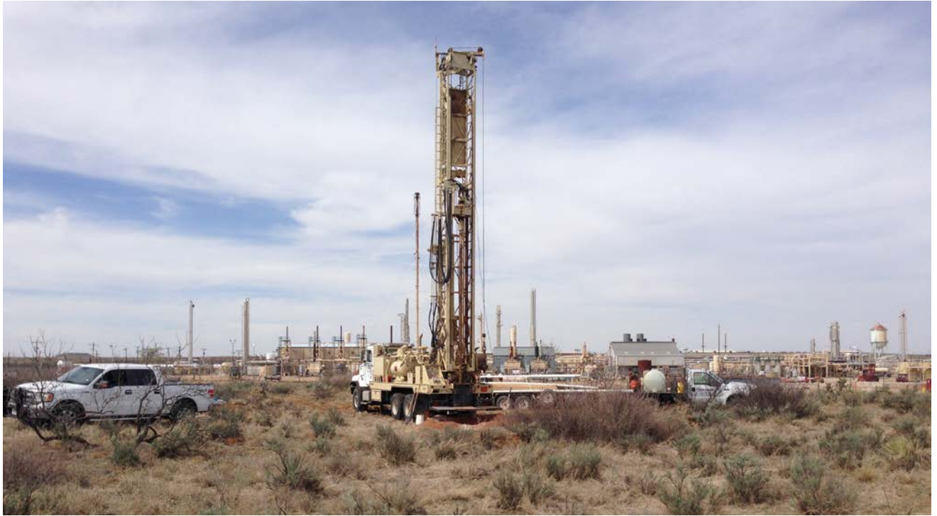
Shallow and Deep Drilling
