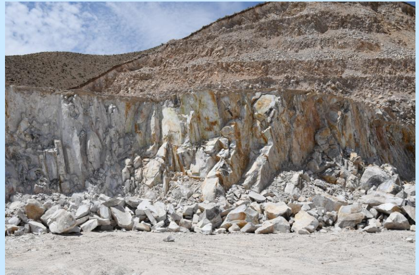
Debris at base of quarry wall.
